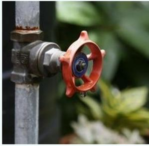
What does exercising a valve entail? Exercising a valve is the process of turning the valve on and then off a few times each year. This keeps the mechanism working and keeps it from “freezing up.” Caution should be used when exercising old valves. An old valve (as seen on the right) could stop in the “open” position but then might not close again. Also, a valve might also stop in the “closed” position but then it might not reopen leaving you with no water inside your home. If this
